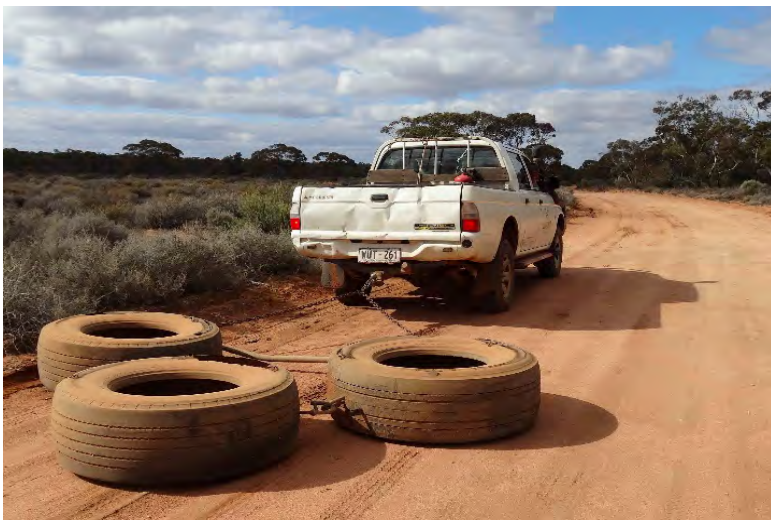
Tyre-dragging is used as an adjunct to grading the tracks.
