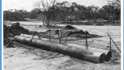
'Bob's Bridge' involved the utilization of a number of secondhand items including dam inlet/outlet pipes from Picnic Dam and Mt Gambier stone bricks from the old Moranvale Homestead
