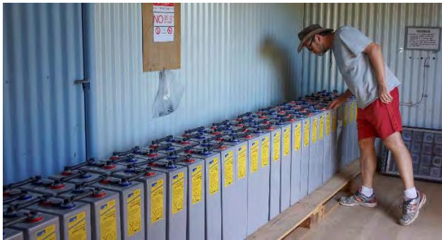
Ranger Peter Struik, inspecting the new gel batteries in the solar power system's battery shed.
