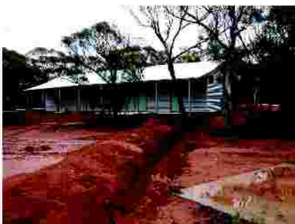
Trenching for water and power to the new accommodation block.
