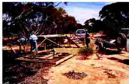
The team erecting pre-fabricated hide sections at Whistler Tank.
